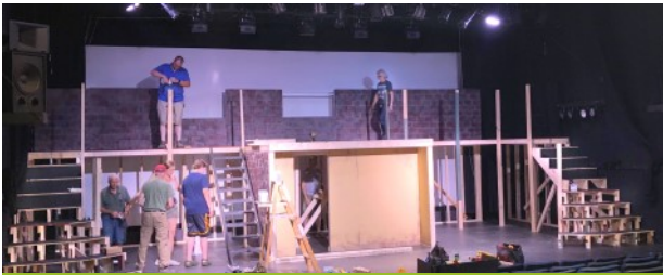
Volunteers erecting the two story set for Sweeney Todd July 2022
